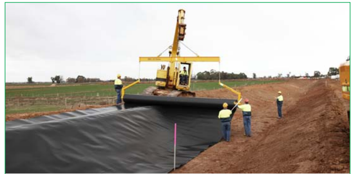
Plastic lining (HDPE) of a canal
