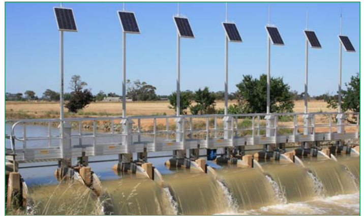
Automatic flow regulating gates
